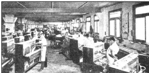
Above: Beale's Piano Factory, Trafalgar Street, Annandale, in 1902. Octavius Beale began operating from the Annandale complex in 1893. (SM, 18 January 1902) Below: Craftsmen assembling pianos at the factory in 1911. Annandale's largest industry employed 560 people in 1920. (ATCJ, 24 May 1911)
