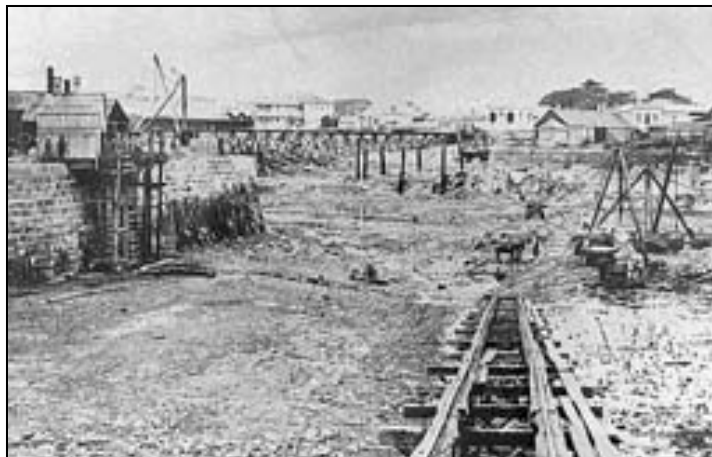
Belmore Basin construction
