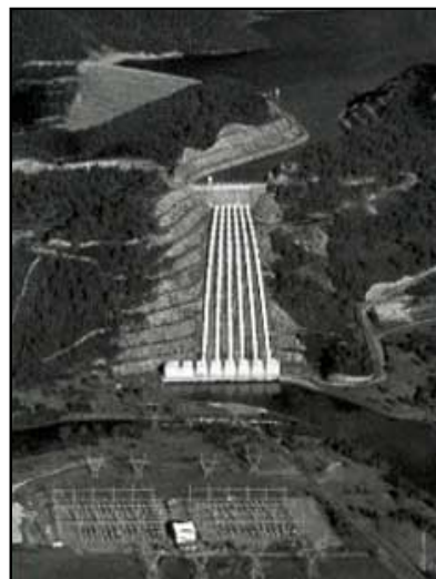
Tumut 3 Power station
