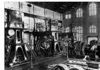
Machinery at Ultimo Power House around 1905. Parsons steam turbine partly visible on the right
