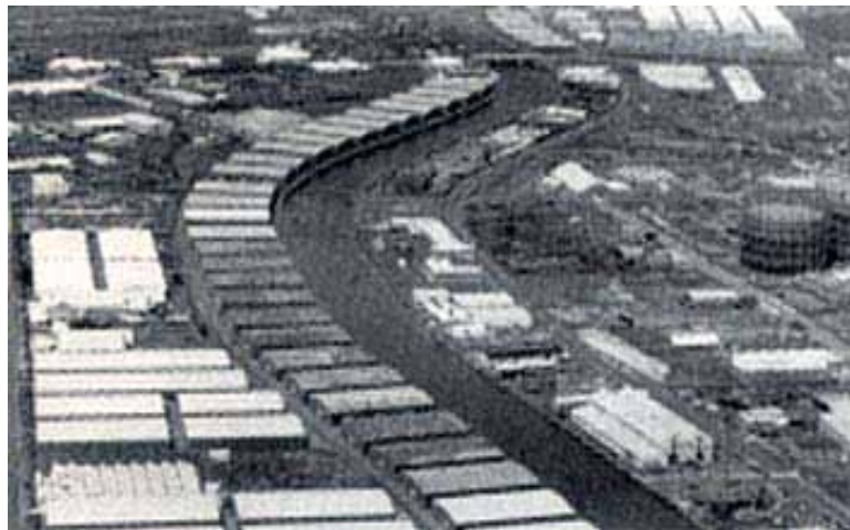
Aerial View of Canal
