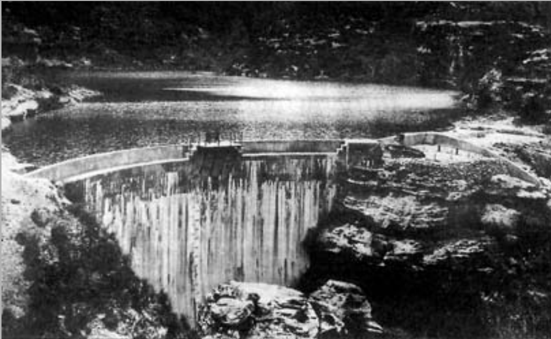
Medlow Bath dam
