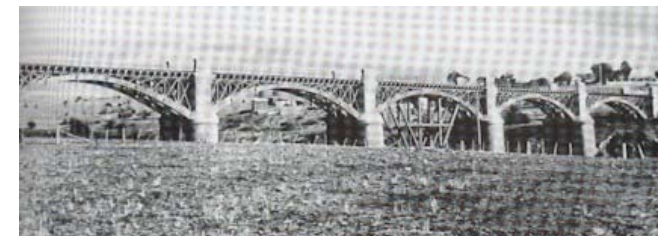
Laminated timber railway bridge, Singleton
