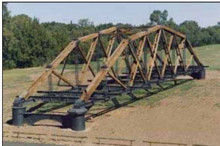
1893 Cowra bridge truss (demolished)
