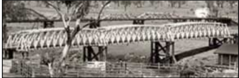
1868 McCallum truss bridge with new McDonald bridge in the background
