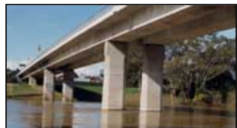
The 1986 (existing) bridge
