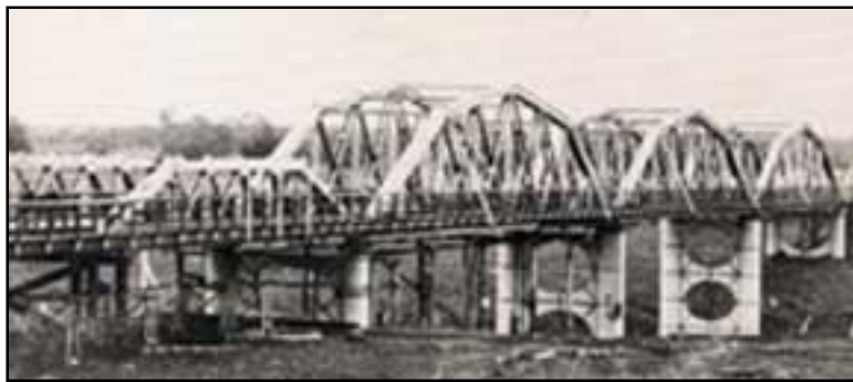
1893 McDonald truss bridge
