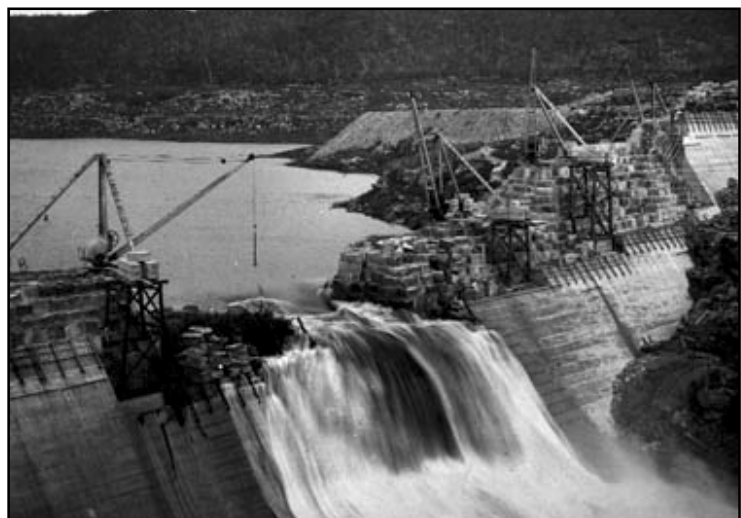
Flood during construction
