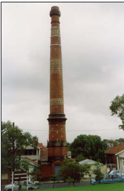
Sewer Vent, Lewisham
