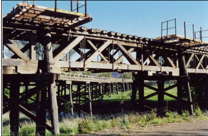
Heritage road and rail viaducts, Gundagai, NSW
